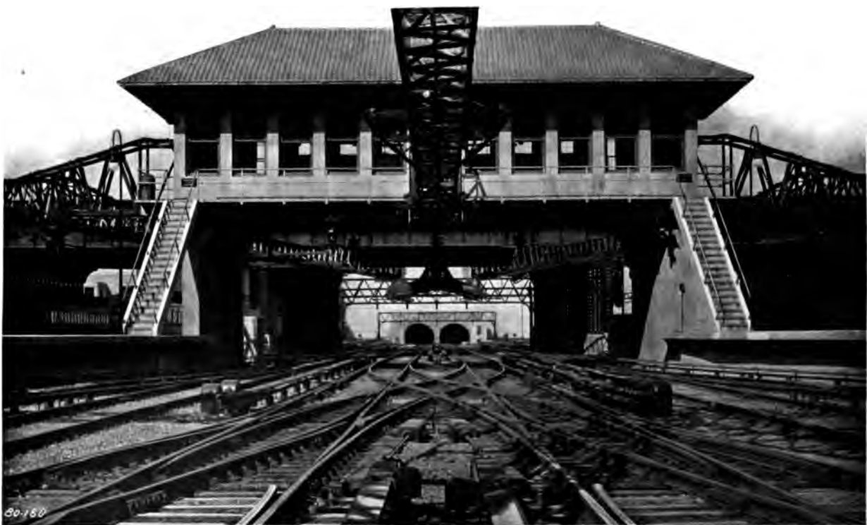
Signal Cabin "A" New York Terminal, Pennsylvania Railroad.
